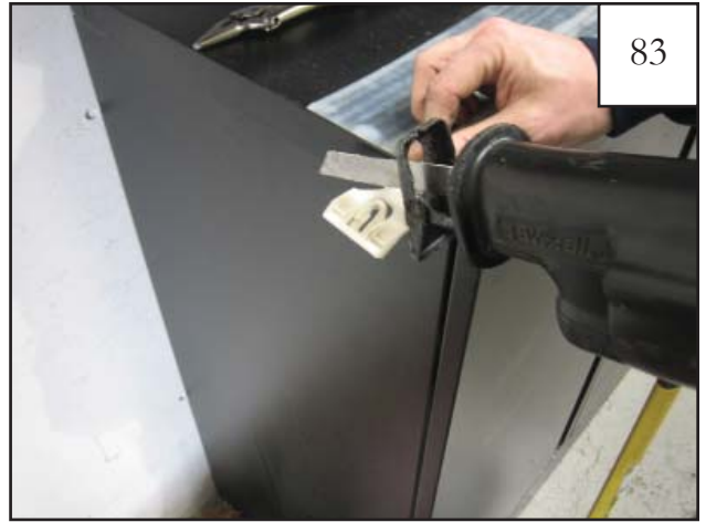
Using a reciprocating saw, cut the cladding clip just below the top section.
