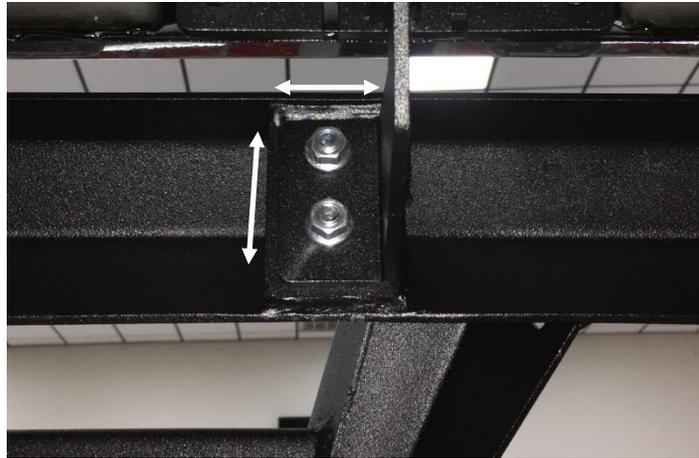
**Step 7:** After final adjustment, torque each bolt to 17 ft/lb – 20 ft/lb.
